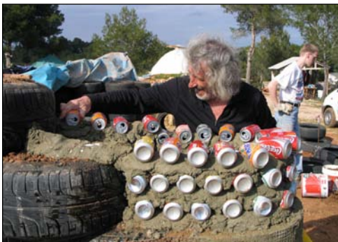
Reynolds constructs a wall out of cans.
